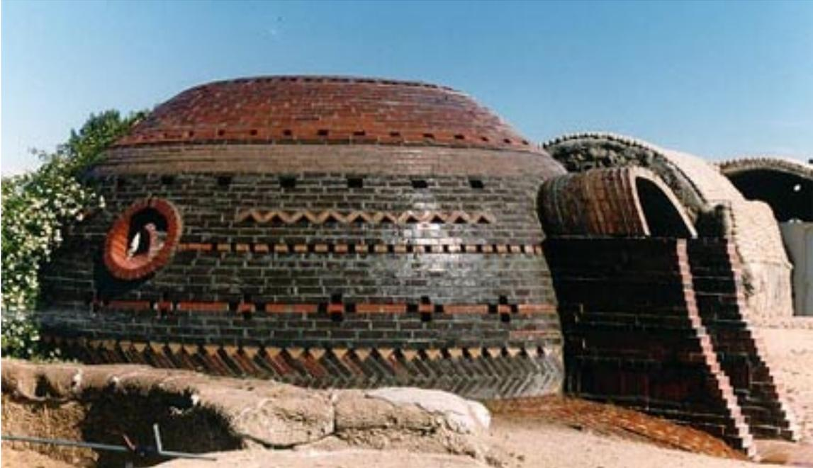
FIGURE14. CalEarth Institute masonry dome, model for lunar masonry vitrified in situ.
